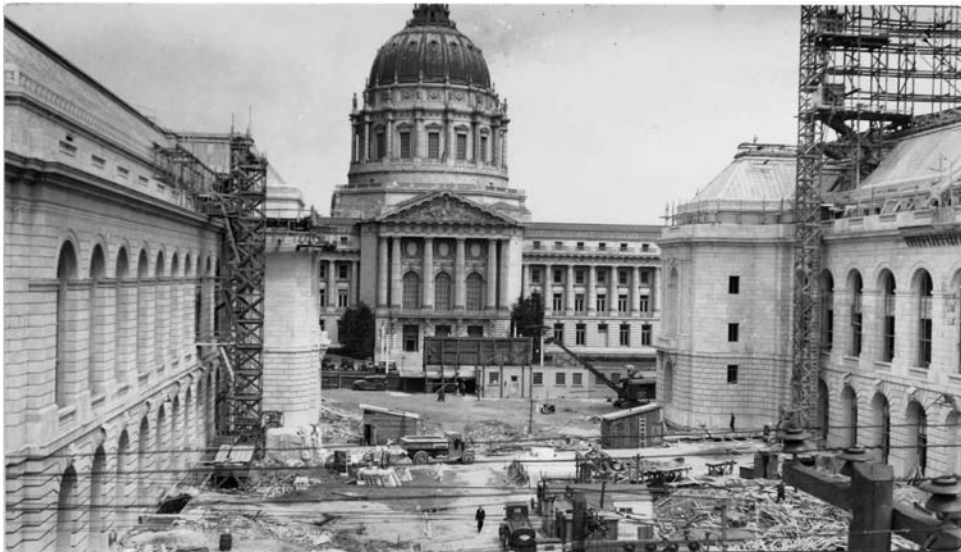
War Memorial Opera House on the right and Veterans Building on the left: construction photo. The courtyard between the two buildings offers a view of City Hall.
