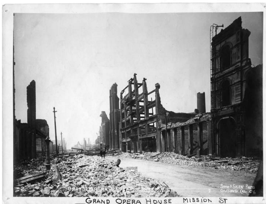
Remains of the Grand Opera House at Third and Mission Streets, destroyed by the fires following the 1906 earthquake.
